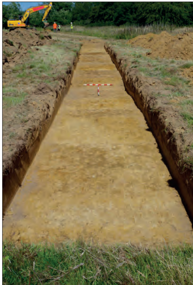
Plate 52: Area vi, Trench 419, viewed from the southwest
