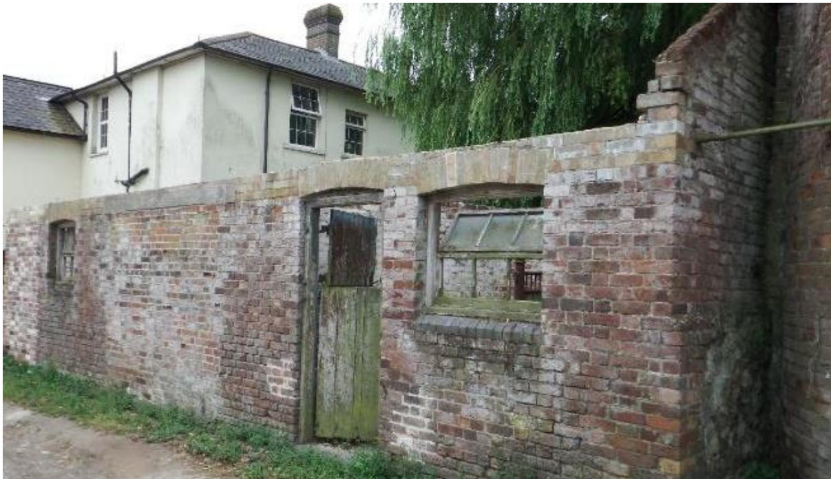
Plate 23: Storage and stables at Barrow Hill Farm
