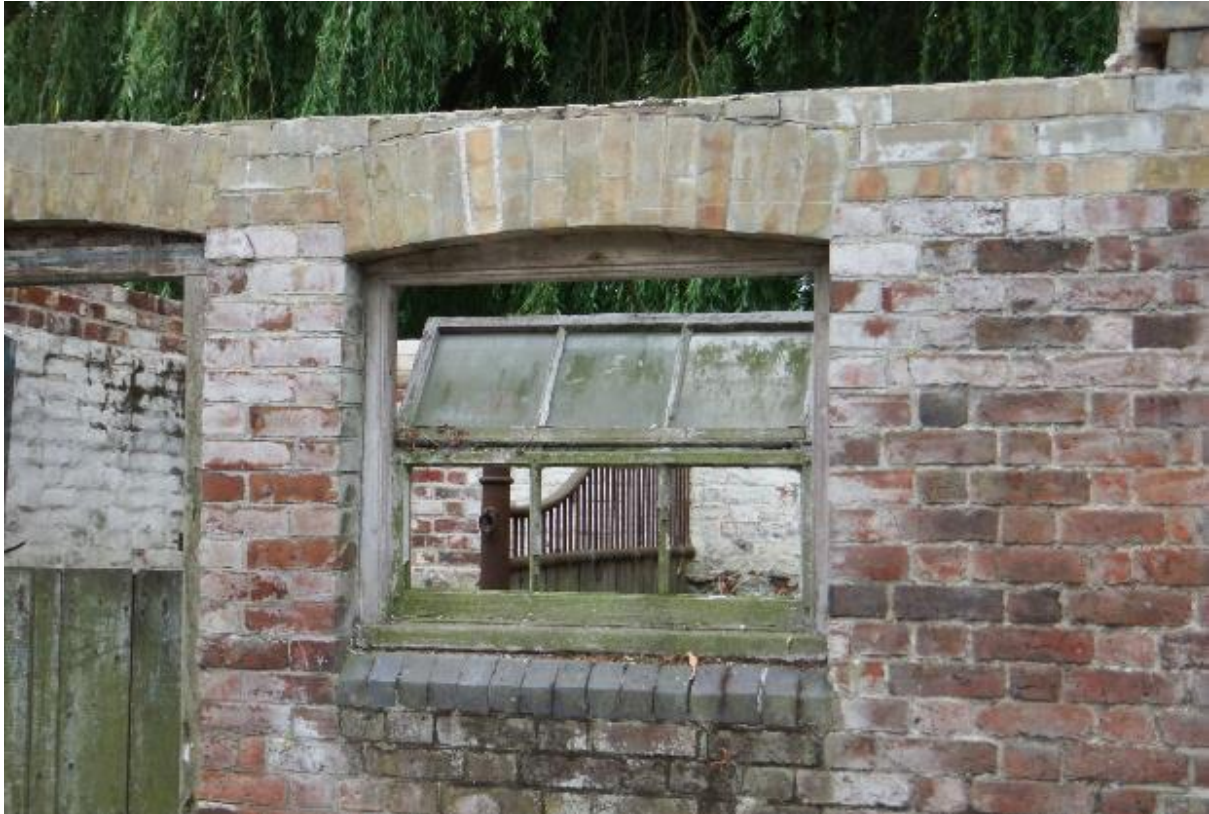
Plate 24: Stables at Barrow Hill Farm
