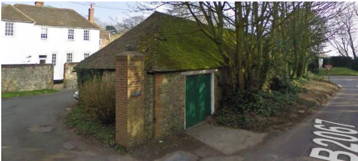
Plate 67: Outbuilding at Bell Vue ( WS6 ) looking south-east (Google Street View 2009)
