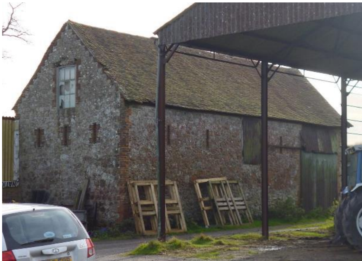
Plate 72: Mid-19 th century ragstone barn with red brick quoins and detailing to the west of the Barn (WS8).
