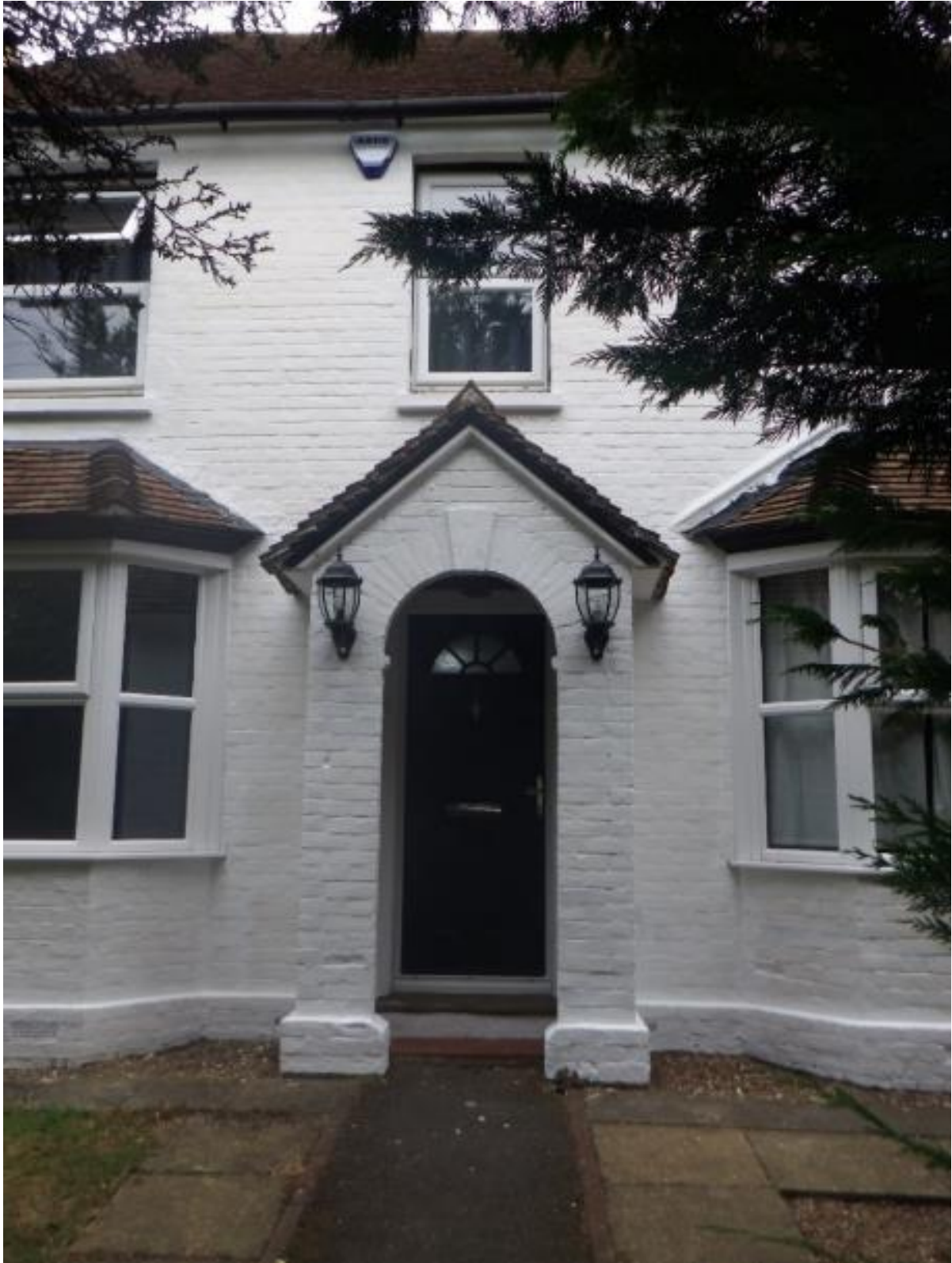
Plate 30: Farmstead South-East of Railway Cottage (BH17) looking east
