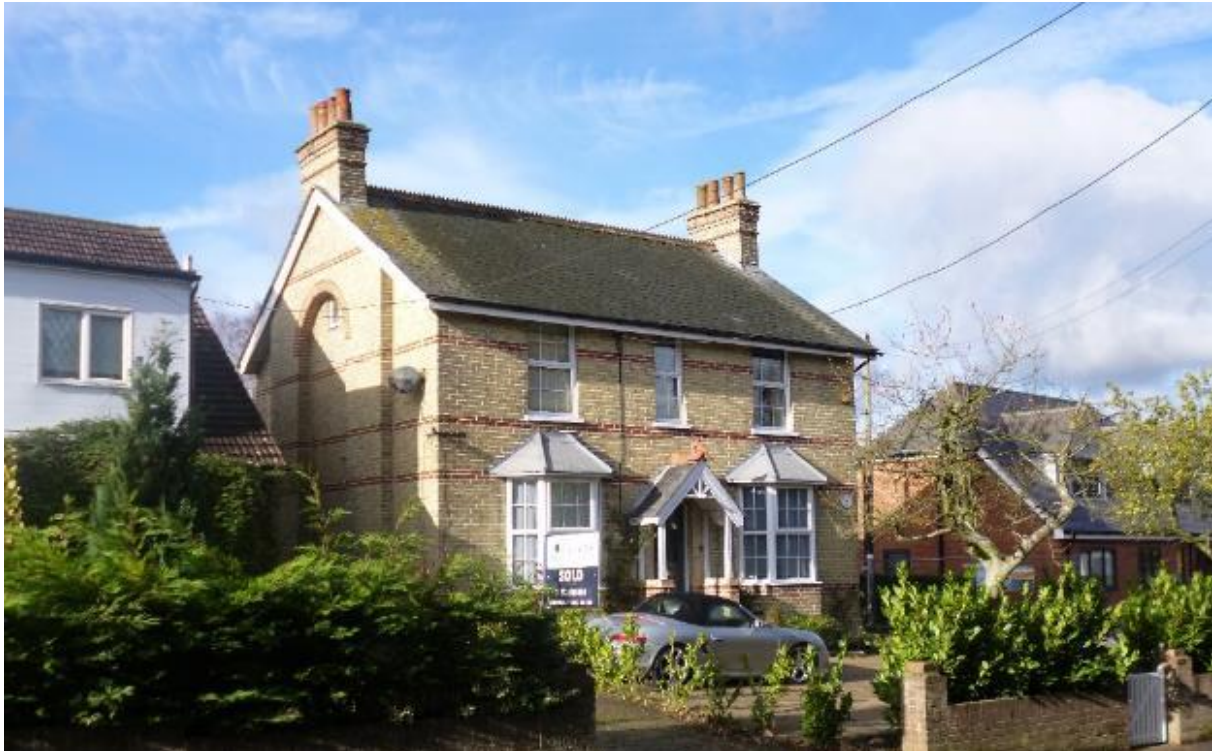
Plate 54: Grove Bridge House (WS22) looking north-west
