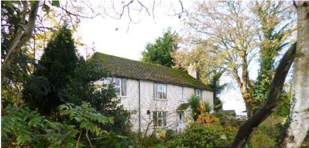
Plate 43: Humble Bee Cottage looking west
