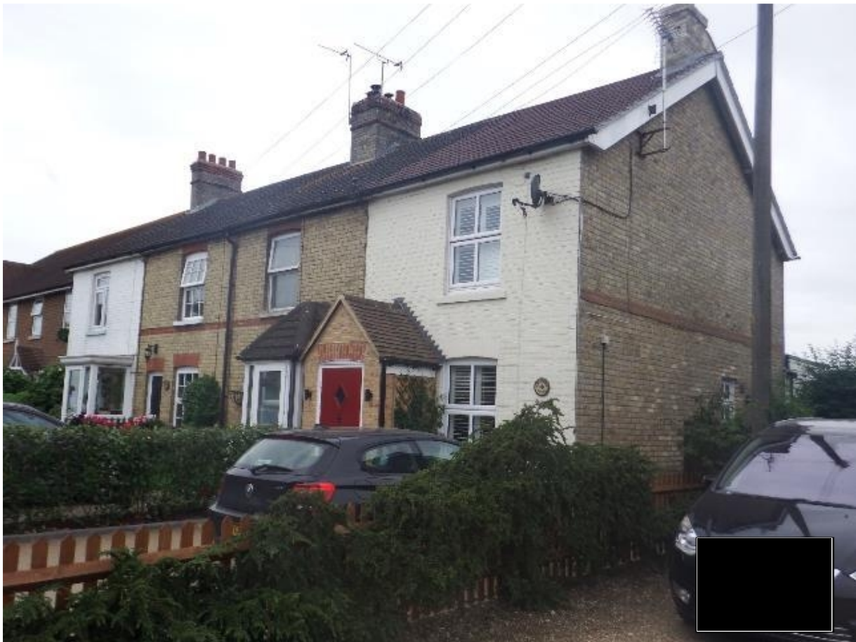
Plate 51: St Johns Villas ( WS25 ) looking south
