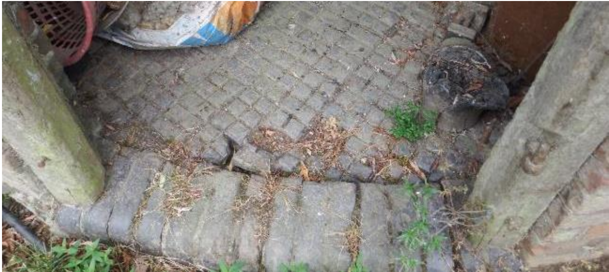
Plate 26: Floor of oast house at Barrow Hill Farm
