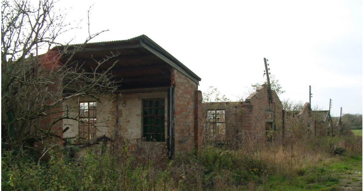
Plate 3: Surviving fixtures at RAF huts west of Otterpool Lane.
