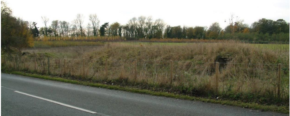
Plate 5: Air raid shelter/bunker at Port Lympne
