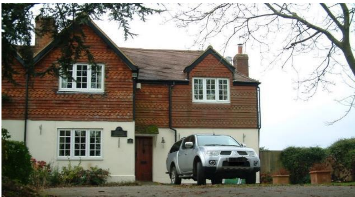
Plate 62: Northern semi-detached cottage Harringe Cottages (WS18) looking west
