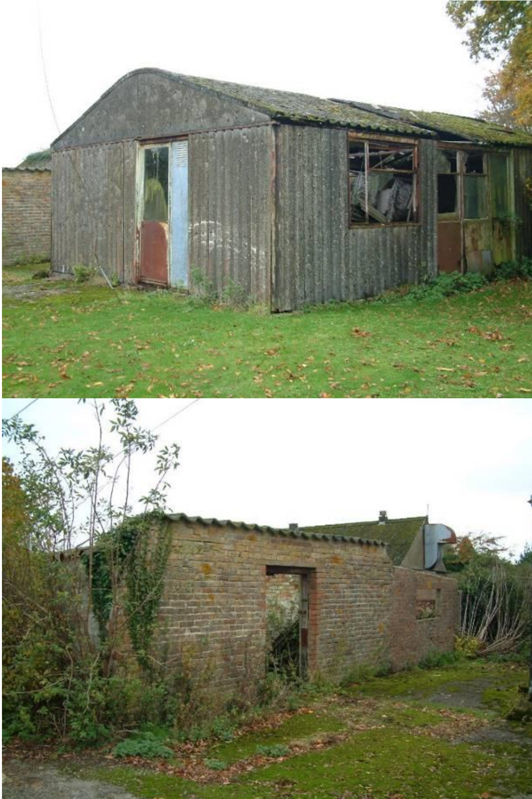
Plate 13: Two of the possible surviving structures from the WWII munitions store.
