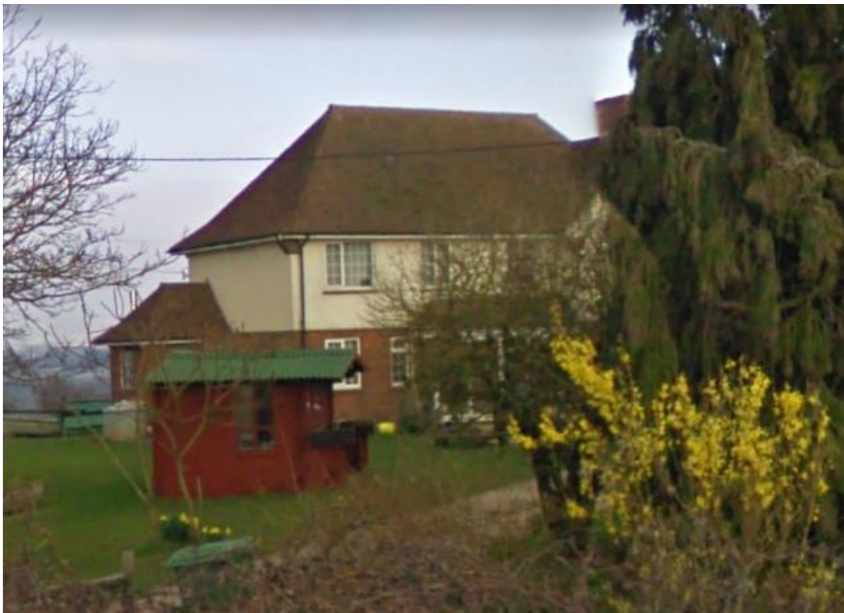
Plate 21: Harringe Court Farm House, looking north-east (Google Street View 2009)
