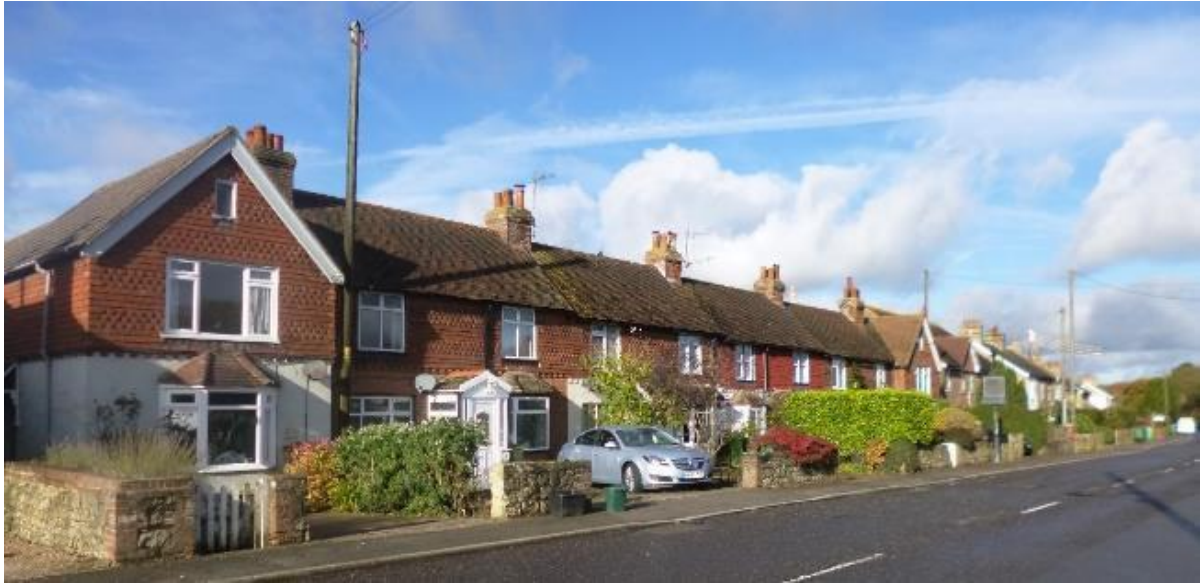
Plate 50: Oak Cottages (WS5) looking north-west
