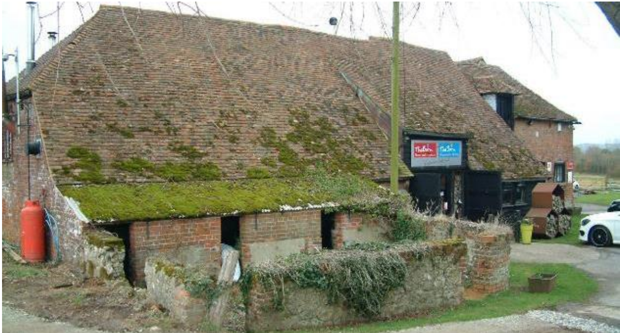
Plate 69: Medieval Barn at Otterpool Manor (WS8) viewed from the southeast.
