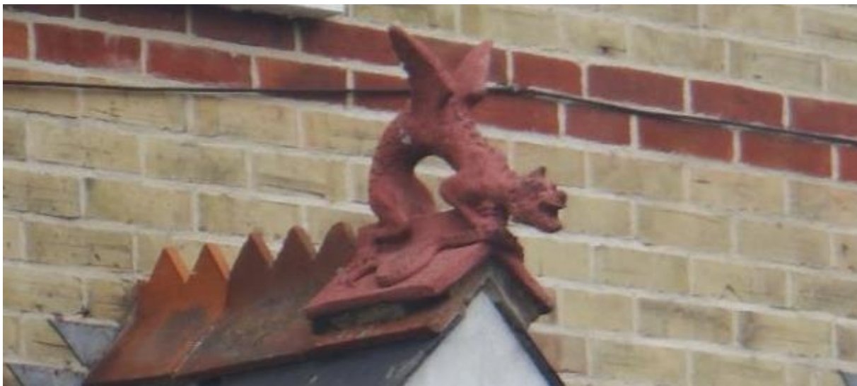
Plate 55: Terracotta dragon on porch of Grove Bridge House (WS22)
