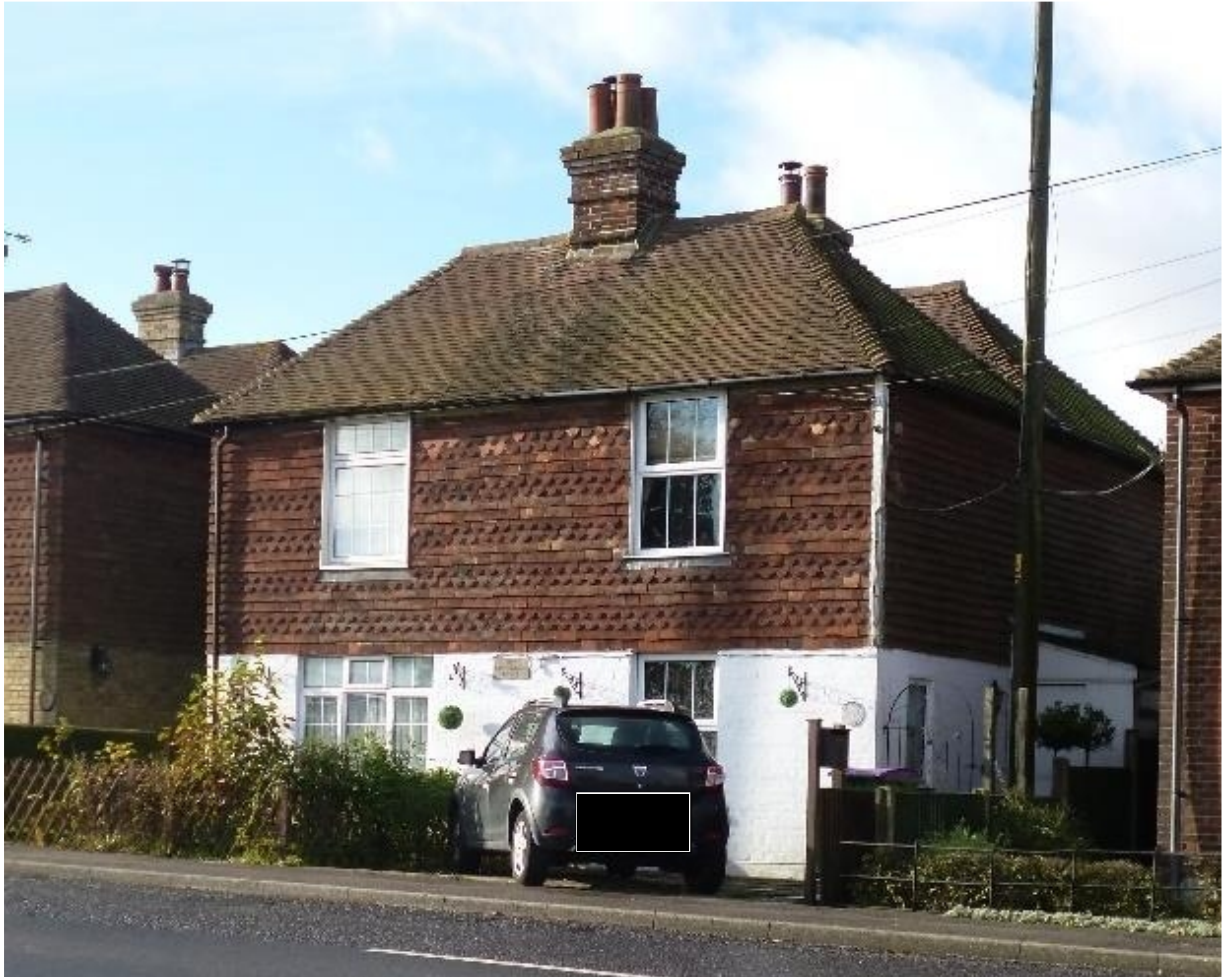
Plate 46: 1 and 2 Ivy Cottage ( WS5 ) looking south west
