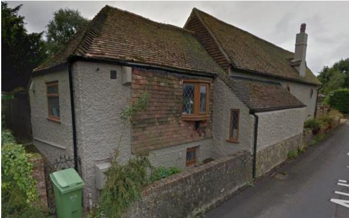
Plate 38: Newell Cottage, Aldington Road looking south-west (Google Street View 2017)
