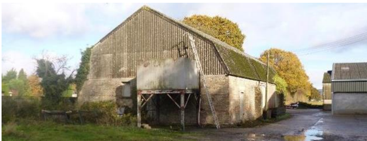
Plate 29: Barn at Barrow Hill Farm ( WS10 ) looking north-east
