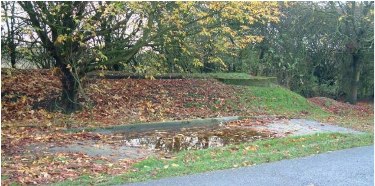
Plate 6: Bunker and concrete wheel wash/former weigh bridge at Port Lympne
