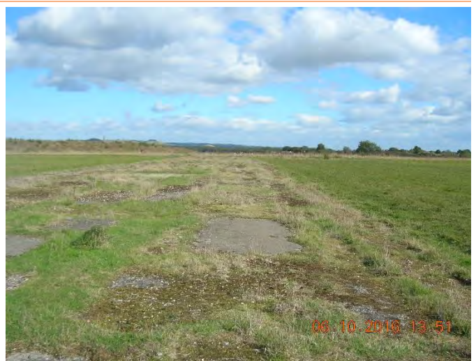
Photo 18: Former taxiway at Lypne Airport
