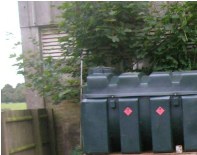
Photo 7: Fuel storage area at racecourse
