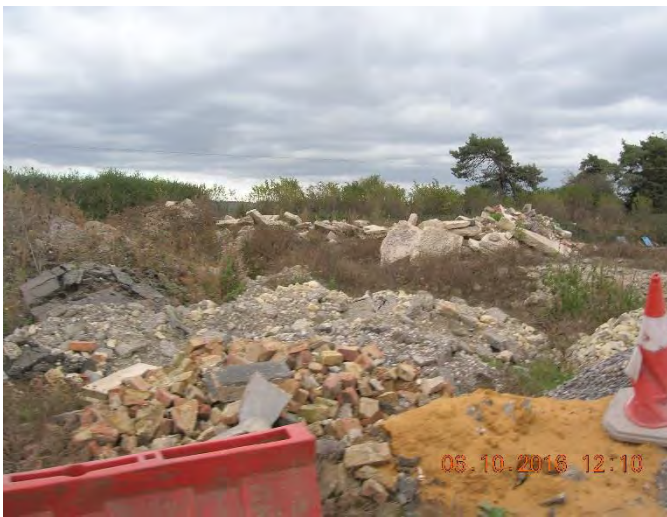
Photo 15: Waste and stockpiles at lorry park
