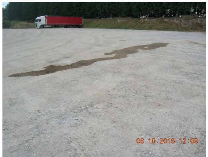
Photo 14: Fuel/oil spillage at lorry park
