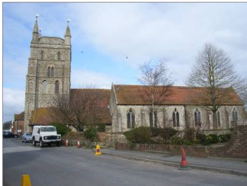
St Nicholas' Church from the south, showing Norman tower and nave (left), and Decorated Gothic aisle and chancel (right)
