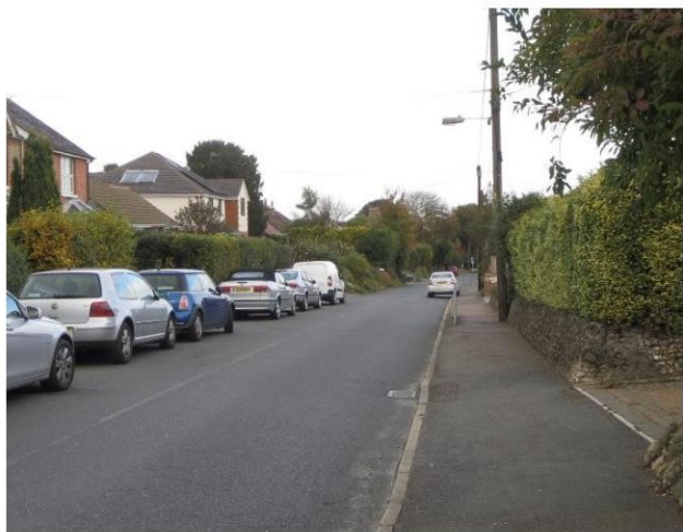
Photograph 16 Stone Street North-bound, through Lympne
