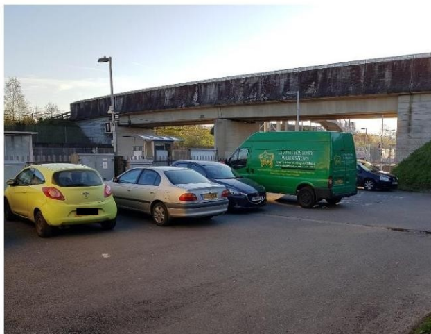
Photograph 7 Westenhanger Station Car Park
