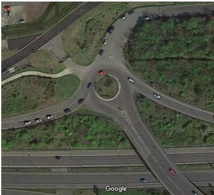
Figure 38. M20 eastbound slip roads / A20 Castle Hill Bridge
