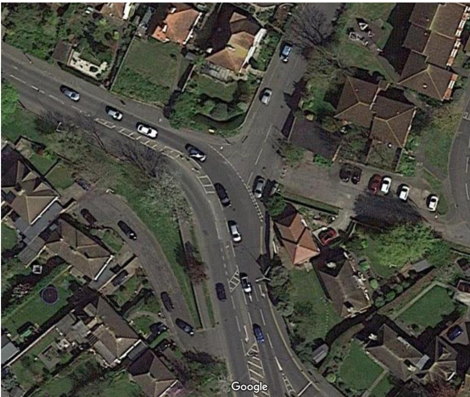
Figure 53. A261 London Road / Barrack Hill
