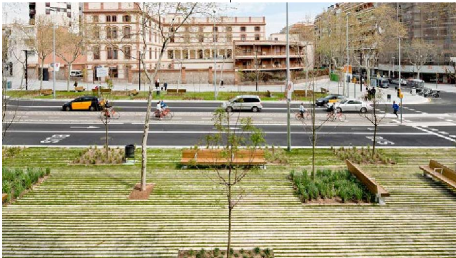
Permeable paving and rain gardens on Pg. de St Joan Boulevard, Barcelona Image credit: Adrià Goula
