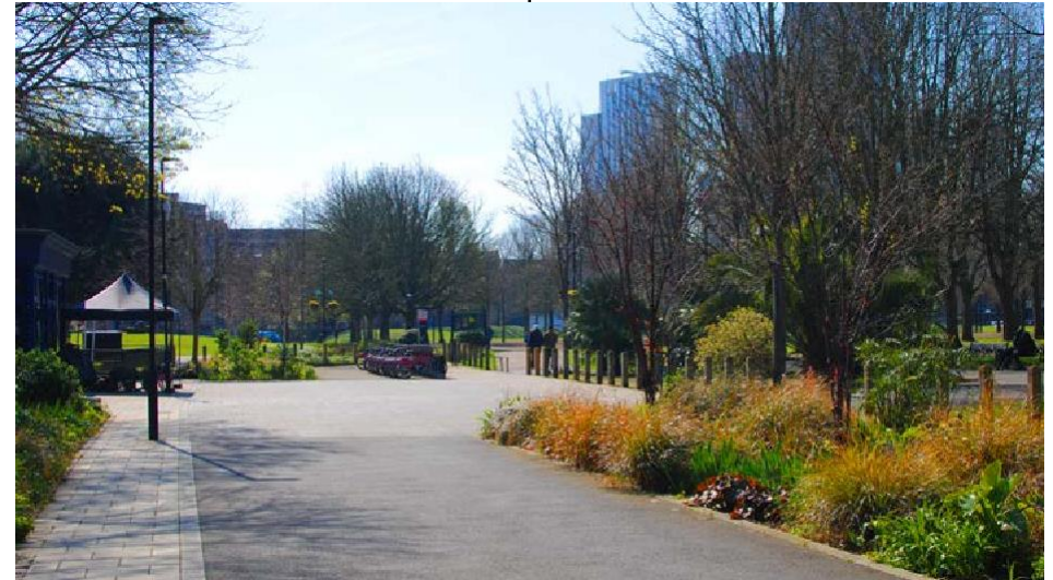
Rain gardens providing greenery and sustainable drainage in Vauxhall, London
