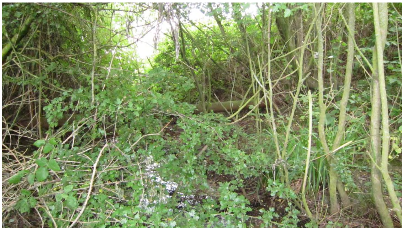
Figure 22 Disused existing metal rising main (220mm outside diameter) at the western edge of the racecourse lake
