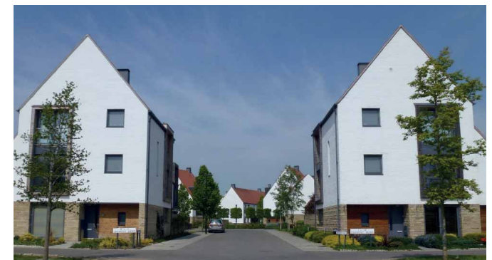
Fig. 5.12: Gateways may be local in character: here at Derwenthorpe the two strong gable ends create a memorable approach to this cluster of homes
