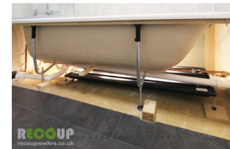
Waste water heat recovery examples from left to right: Horizontal – underneath bath or shower tray
