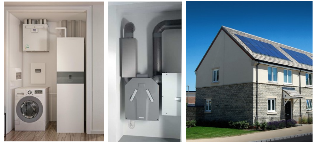
Technology that drives down energy consumption is easily available. Designers and contractors must however allow for these systems early-on in scheme conception and pay close attention to their installation, commissioning and maintenance. Allowing space on floor plans from an early point in design is crucial. The above images show the integration of (from left to right) an individual heat pump, a mechanical ventilation system with heat recovery, and roof mounted photovoltaics.
