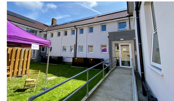
Ross House in Folkestone, the council's first 'net zero' enabled residential block
