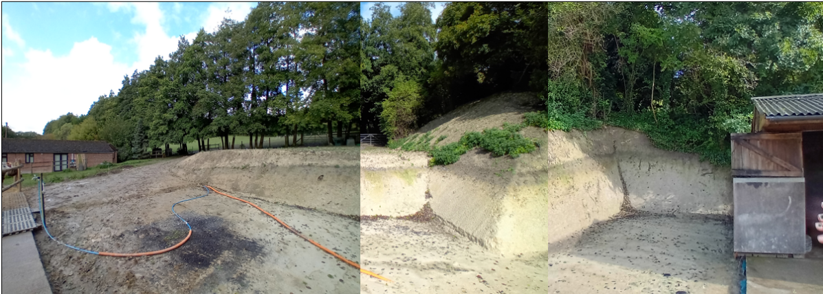
Figure 6: Existing stables and groundworks
