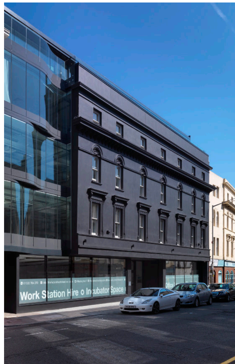
The Workshop, Guy Hollaway Architects © Charles Hosea
